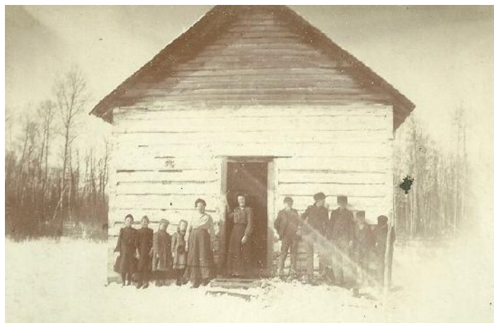
Log School, District #8, Frohn Township [BCHS-1481].
